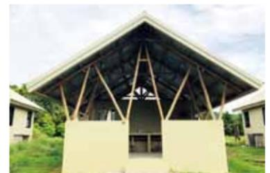
Figure 6. Actual Photo of the Constructed Social Activity Building, featuring Cement Bamboo Frame Technology
