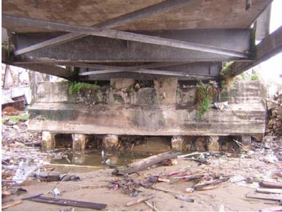
(a) NW abutment with visible piles
