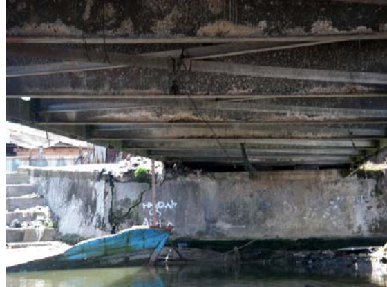
(b) SE abutment
