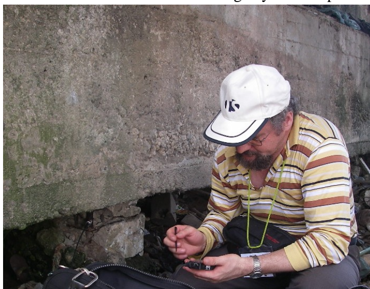
Figure 4. Measurement on the breakage and corrosion state of reinforcing bars
