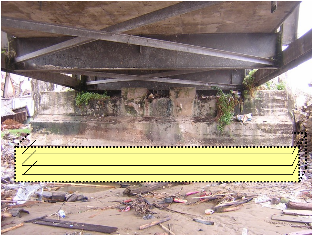
Figure 7. An illustration of casting a reinforced concrete slab around the pile heads of the piers of the abutments.
