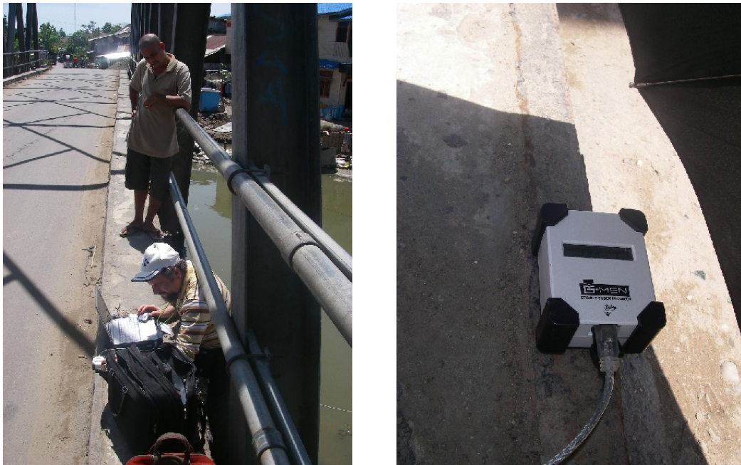
Figure 3. Acceleration measurements of the bridge by a 3-component accelerometer
